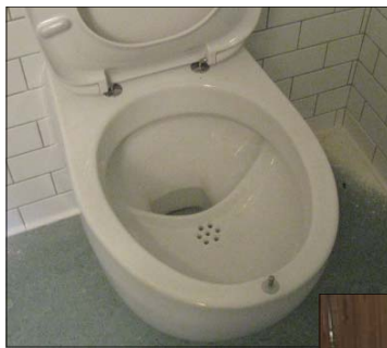
Bellingham's first urine separation toilet...
